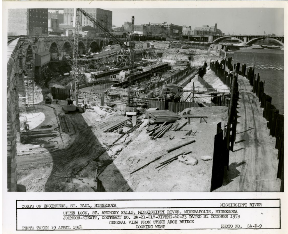
Figure 5-4. Upstream View of USAF During Construction.
