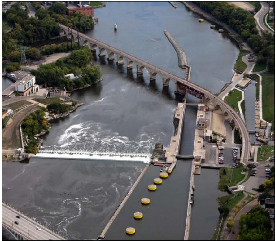
Figure 1-6. Upper St. Anthony Falls Lock and Dam
