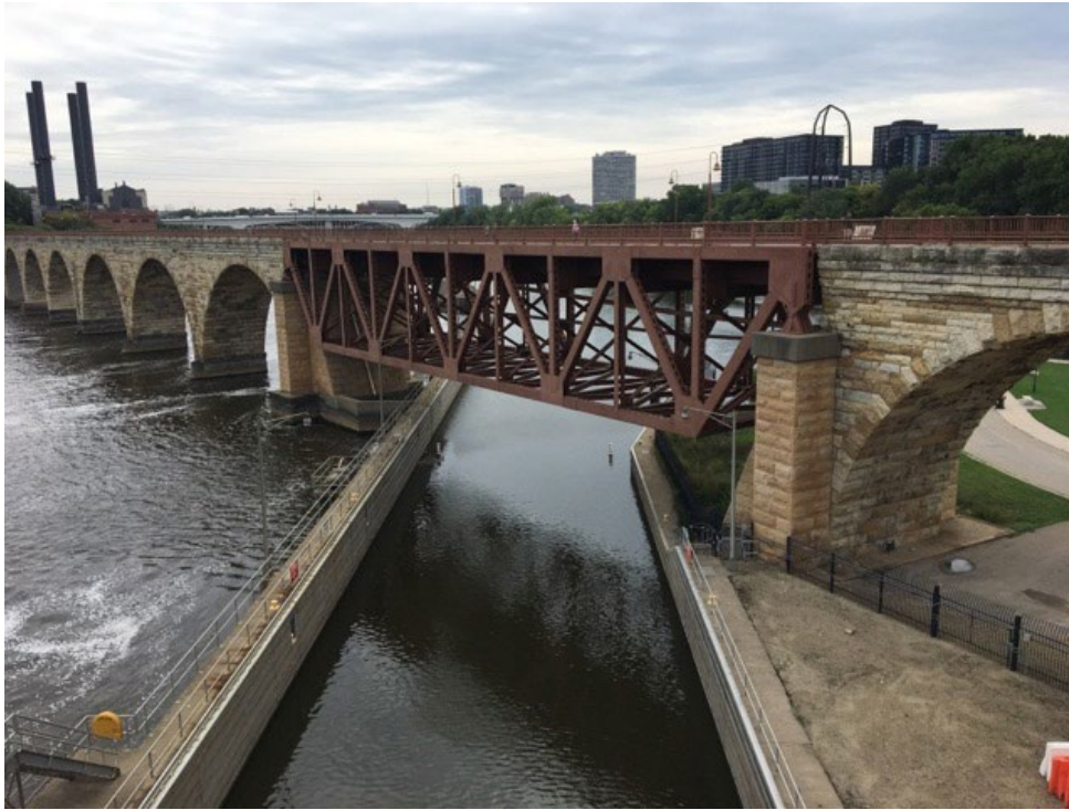
Figure 5-5. Stone Arch Bridge Metal Truss Over Lower Approach to USAF
