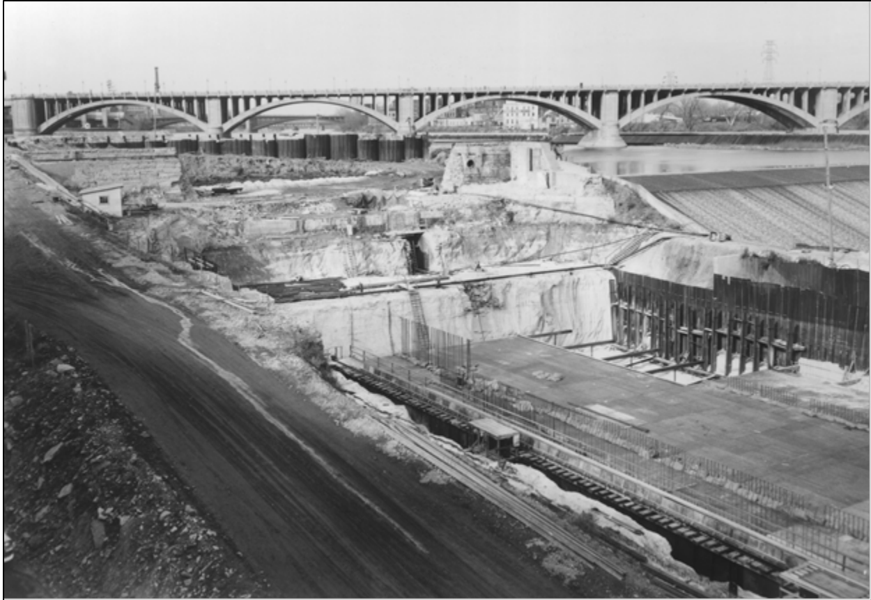
Figure 5-2. Upper Saint Anthony Falls Lock Construction
